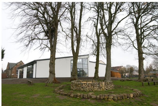
Our extension viewed from the grounds at rear of school
